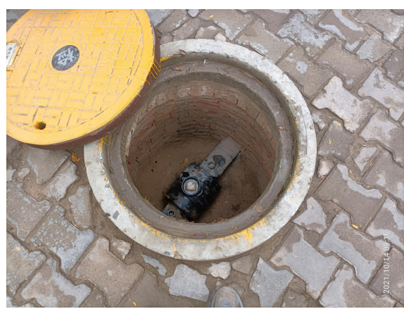
翔凤大桥东侧阀室打开状态 (110°10'33.660", 37°44'59.584")
